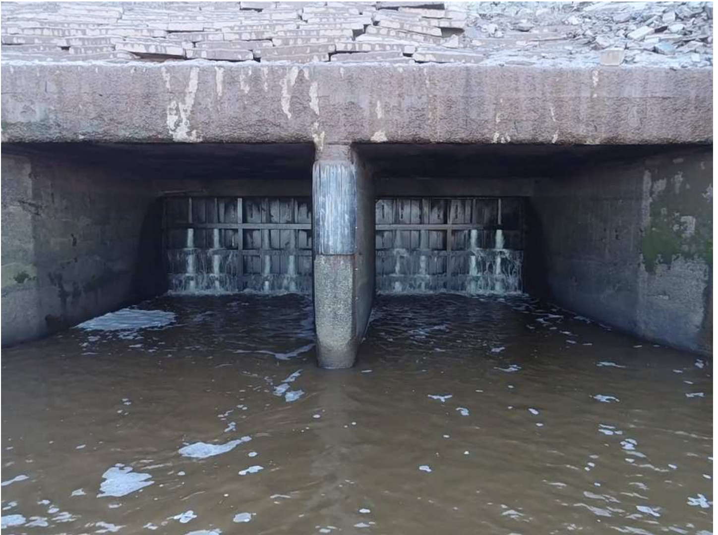
Figure 2: Looking from the ocean at the gates to the Windsor impoundment. Near low tide, an HR2 receiver was mounted a ledge of each gate. At high tide, water rises well above the top level seen in the photograph.
